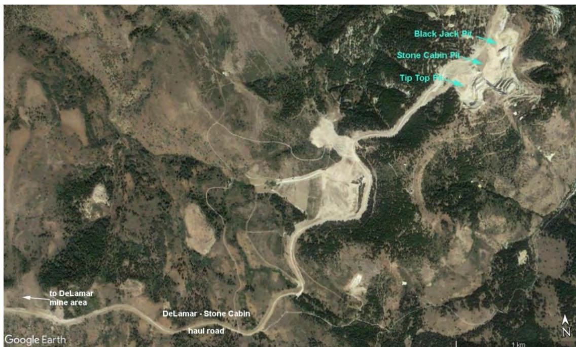
Figure 6-3 Aerial View of the Florida Mountain (Stone Cabin Mine) Area (produced by RESPEC, 2019)
